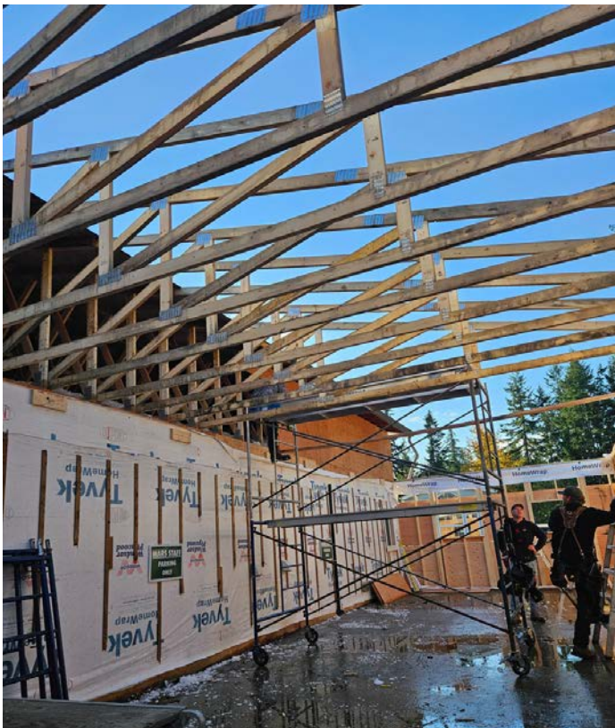
Progress moving fast on the hospital expansion
